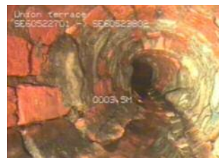
Brick sewer prior to lining
