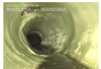
Brick sewer post lining
